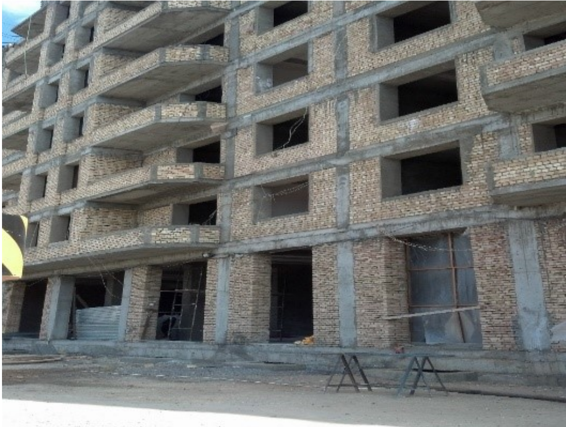
Figure 1. One of the brick multi-storey residential buildings under construction in Samarkand.
